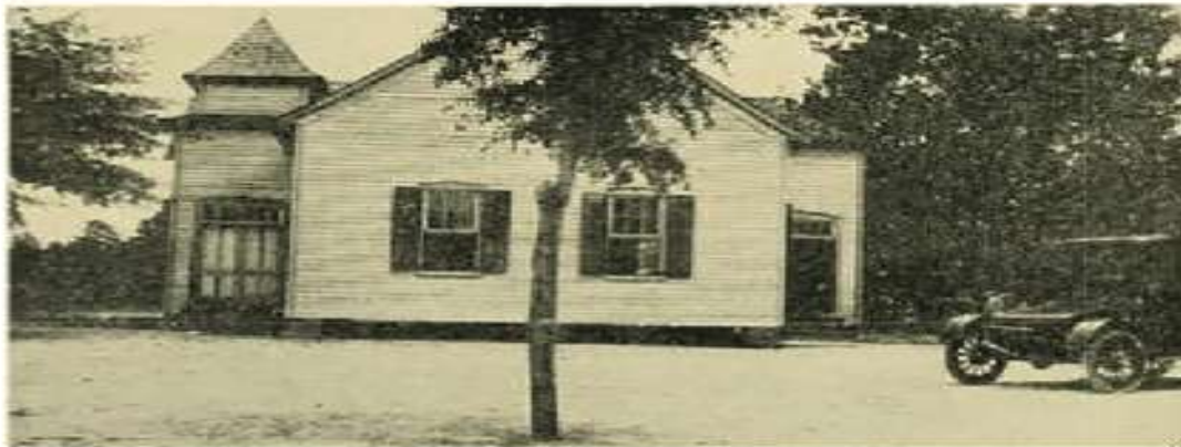
Fig. 2.16. St. Nicholas Lutheran Church, 1924. In 1910 the church moved to its fourth—and present—location on land given by Charles David Loadholt. The cemetery was also established in 1910. Until 1937, the building had two front doors. Courtesy Robert Edward Connelly, III, and Anna Katherine "Kathy" Black Henson.
